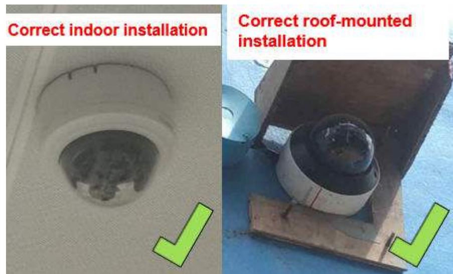
Figure 3-32 Correct installation example
