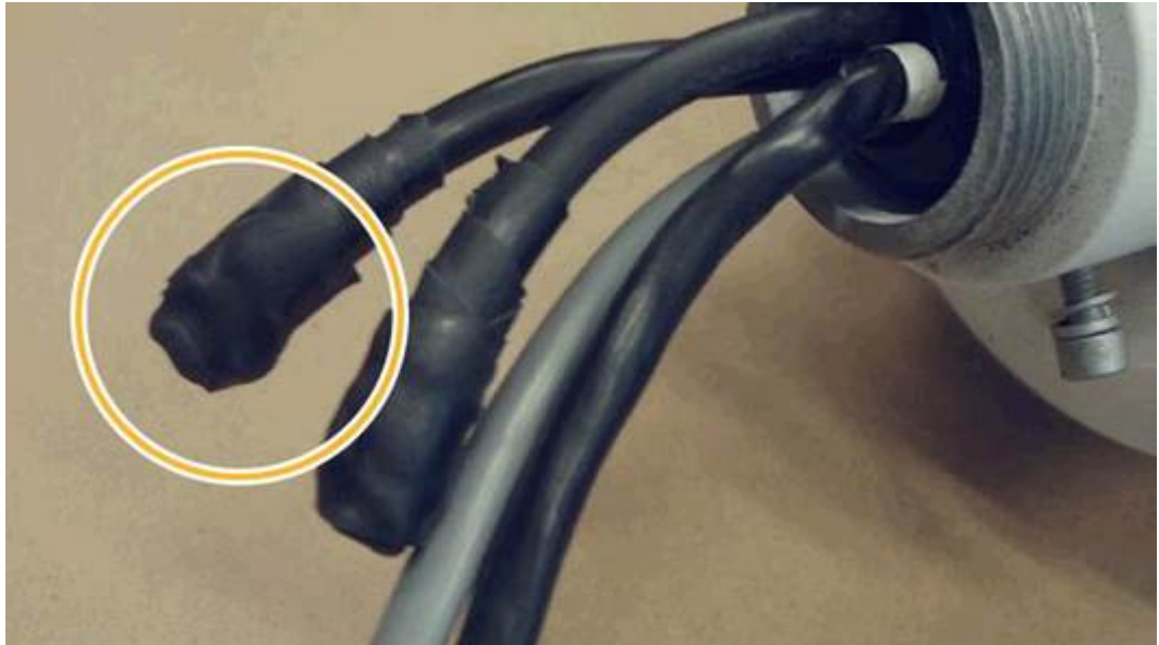
Figure 3-2 Apply waterproof tape on the pigtail
