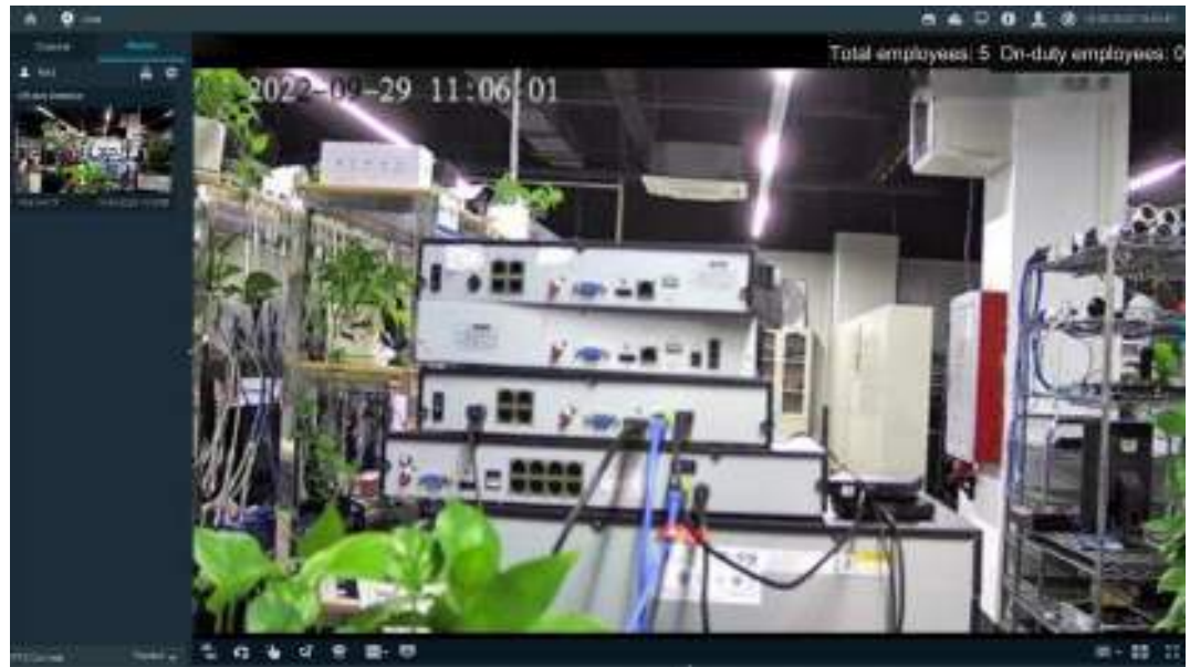
Figure 3-77 Viewing an alarm
